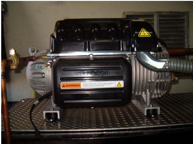
July 2005 Turbocor 120-ton Compressor Installation in the City of Commerce
